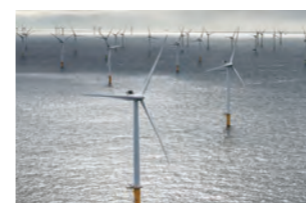
Offshore wind farm
