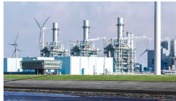
Magnum Power Plant Project in the Netherlands (one of the world's largest 100% hydrogen fired power projects).
