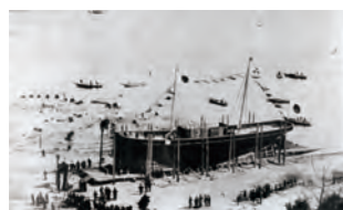
Nagasaki Shipyard & Machinery Works' first steel steamship, the Yugaomaru
