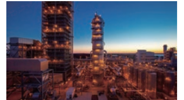
CO 2 capture plant
