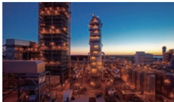
CO 2 capture plant
