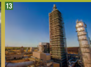
CO 2 Recovery Plant
