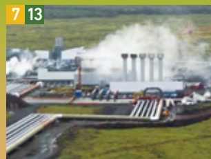
Geothermal Power Plant
