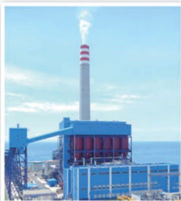
▲ Paiton III Thermal Power Plant
