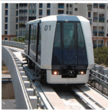
▼ Sengkang/Punggol Light Rapid Transit APM System in Singapore
