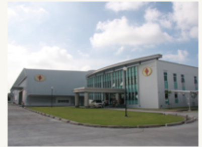
Recently completed EGAT Diamond Service maintenance center for high-temperature components in gas turbines
