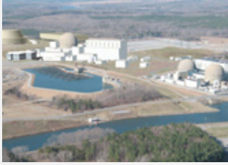
Rendering of proposed US-APWR North Anna unit-3 U.S. Utility, Dominion Virginia Power
