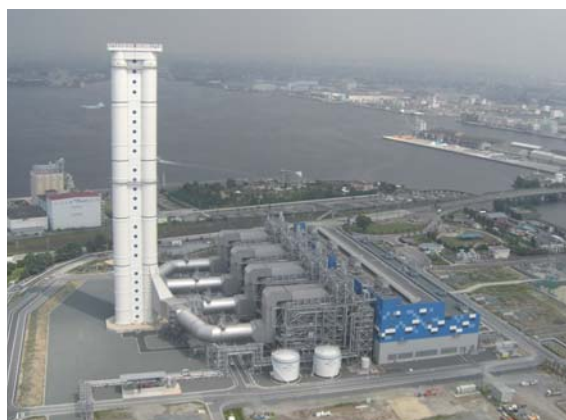
Gas Turbine Power Combined Cycle Plant (Chubu Electric Power Company)
