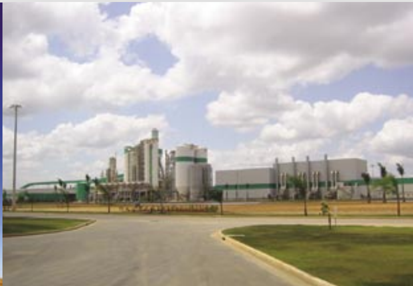
125MW Steam Turbine Plant (Brazil)
