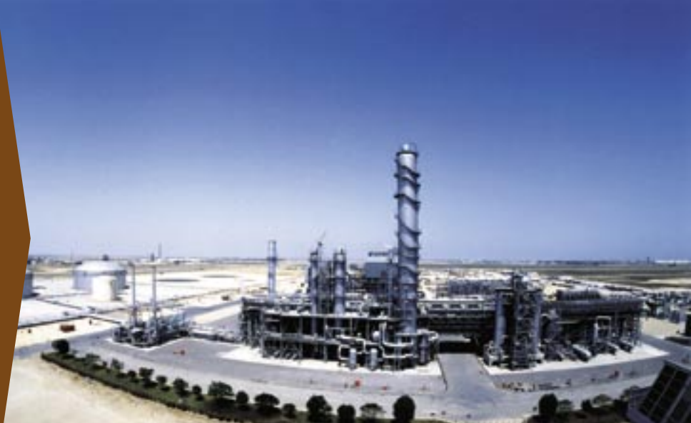
Methanol Plant (Saudi Arabia)
